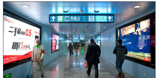
Figure 3-6 Digital advertising displays flush mounted in station wall panel system (Beijing, China).
