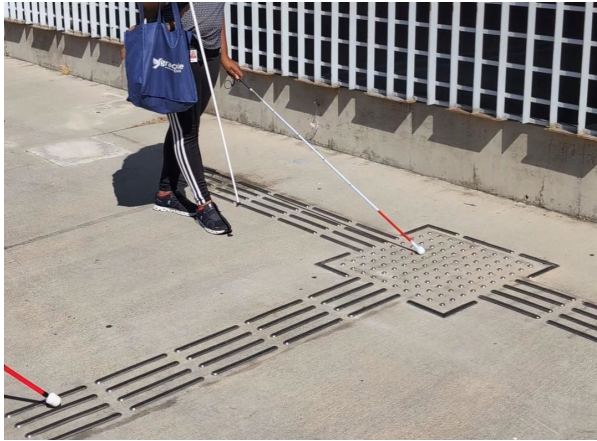
Figure 2-7 Stainless steel tactile wayfinding elements with black non-slip inlays, in a test installation.
