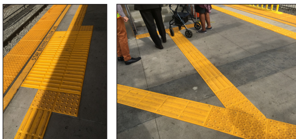
Figure 1-1 Overuse of tactile tiles creates impediments for other station users, confusion between areas of wayfinding and areas of warning, and an inconsistent tactile format that is challenging to navigate (Willowbrook/Rosa Parks Station).
