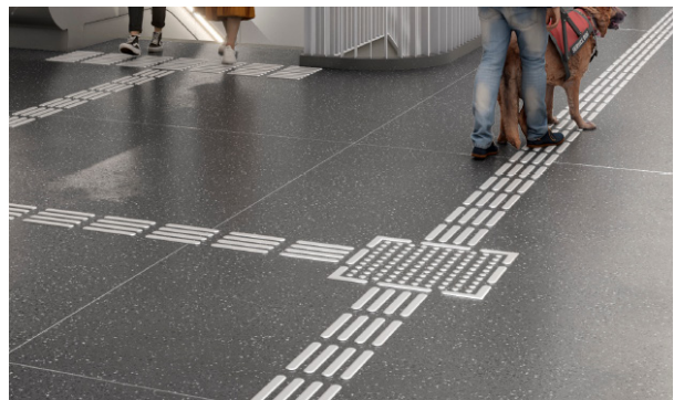
Figure 3-2 Tactile wayfinding concept with four parallel stainless steel bars. Truncated dome array indicates directional pathway change
