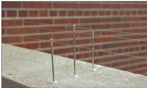
Figure 3-6 Example bird wire system installation.
